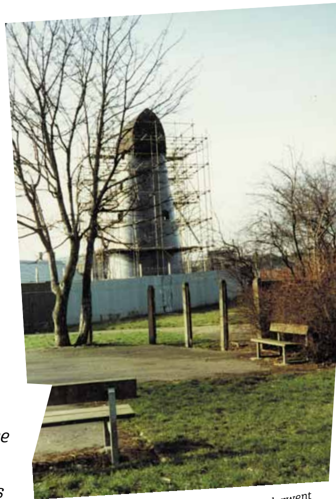
In 1985 the windmill underwent major restoration. Millwright David Nicholls removed the cap, made new sails and repaired parts of the brick tower
