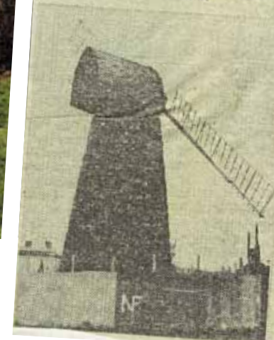
In May 1982 the South London Press reported serious vandalism at Brixton Windmill
