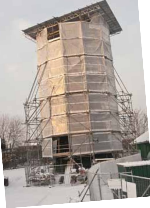
During one of the coldest winters of recent years Brixton Windmill without its sails or cap was wrapped in plastic as restoration work went ahead
