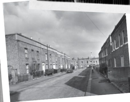
Prague Street, typical of the Victorian terraces near the windmill where Florence Hall and Maureen Lemon grew up. In 1968 these houses were about to be demolished to make way for the new Blenheim Gardens Estate
