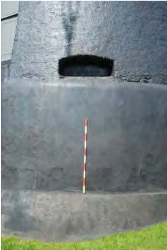
Fig. 37: Photograph of the indented arch (possibly an earlier doorway), on the south-eastern side of the structure.
