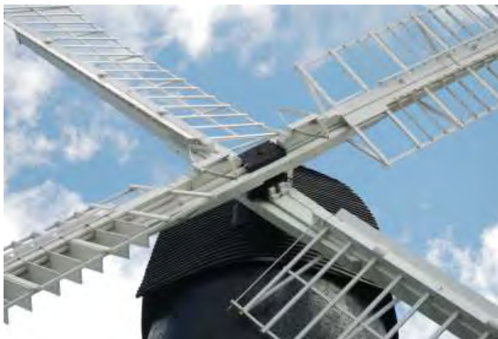
Fig. 52: Photograph of the central part of the sails, showing the stocks and central 'canister'.
