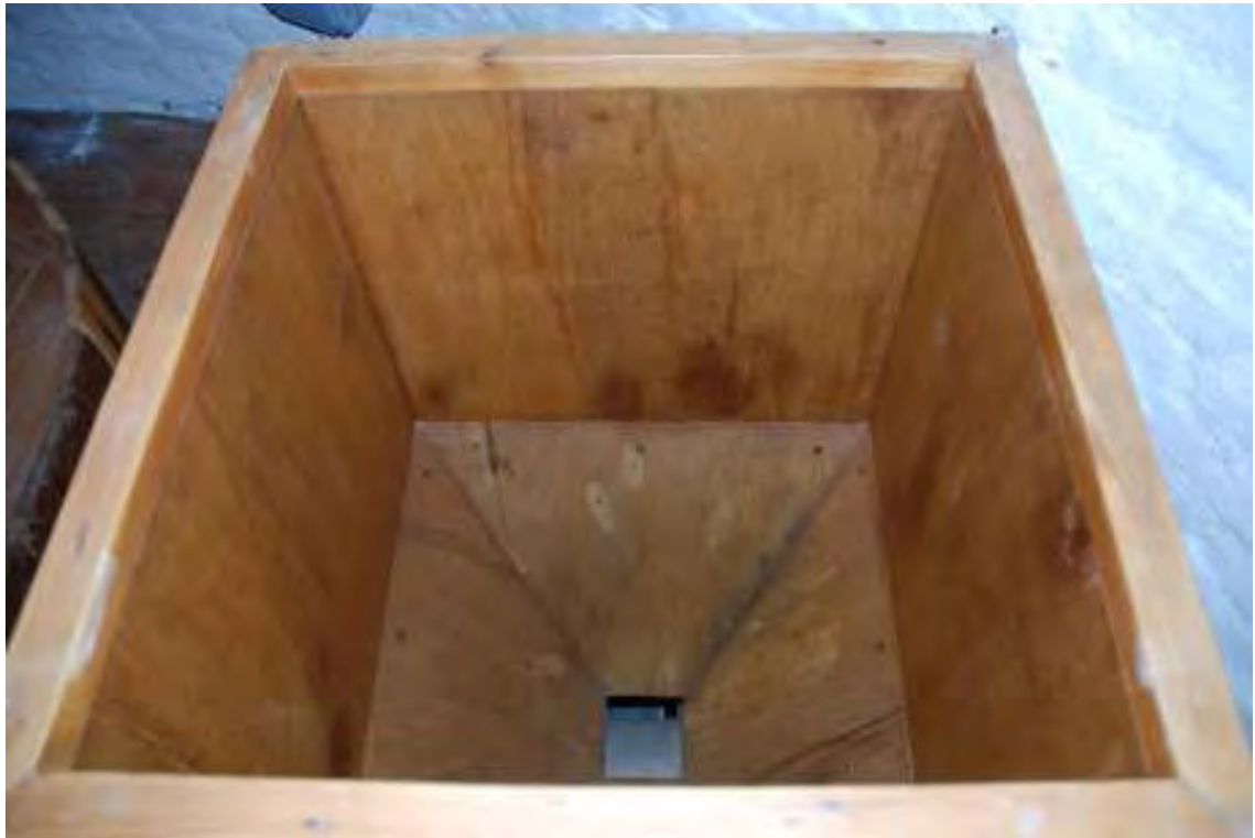
Fig. 77: Photograph of the wooden chute in the northern side of the second floor, not original.
