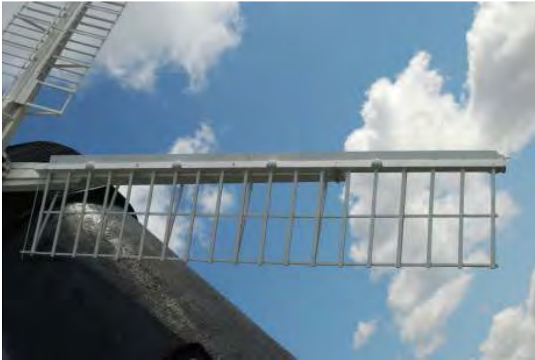
Fig. 49: Photograph of one of the 'common sails' today. The attachments to which the cloth could be attached to (the round fittings) can be seen.
