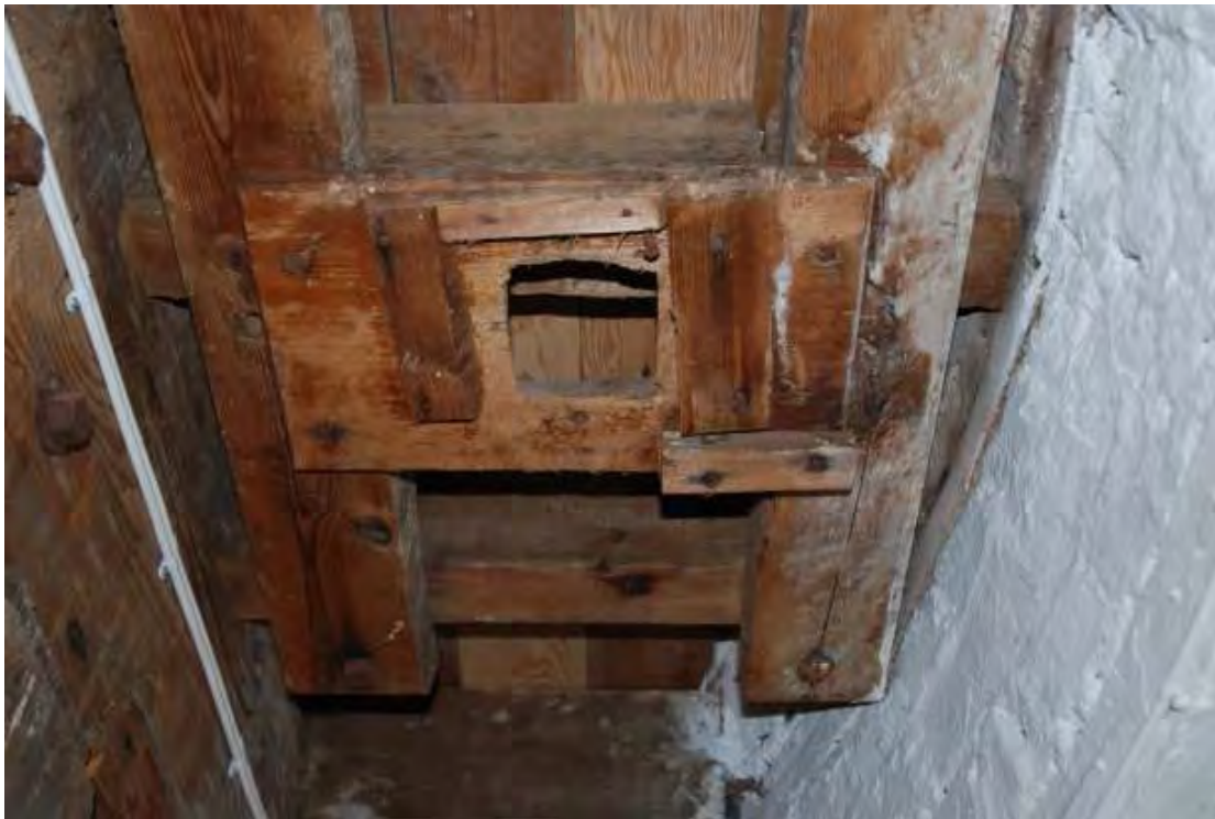
Fig. 79: Photograph of the square base-plate, on which a chute was presumably once attached, on the north-western side of the structure.
