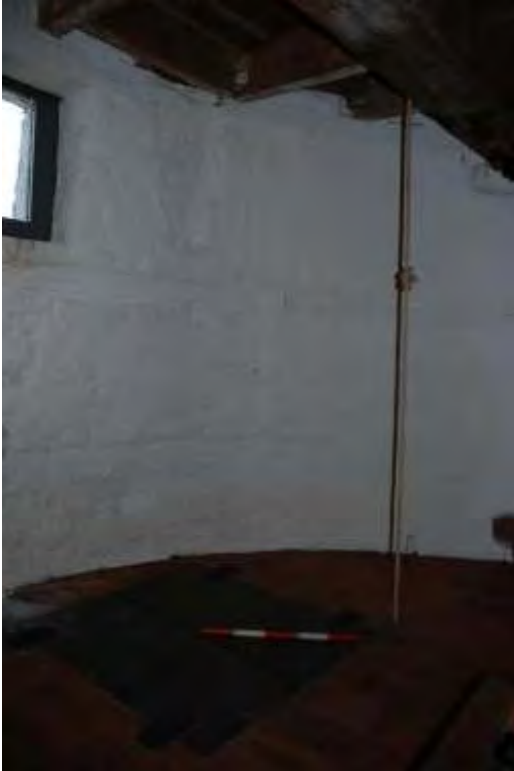
Fig. 59: Photograph of the trapdoors on the third floor (one in the floor and one on the ceiling) - both replaced.
