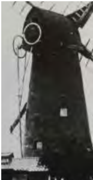
Fig. 45: Extract from a pre-1862 photograph, clearly showing the two wheels which could be operated from the first-floor stage. The one directly at the rear of the cap operated the patent sails (through the striking rod system taken through the windshaft), and the one to the left of this rotated the cap (from Greater London Council 1967 pamphlet).
