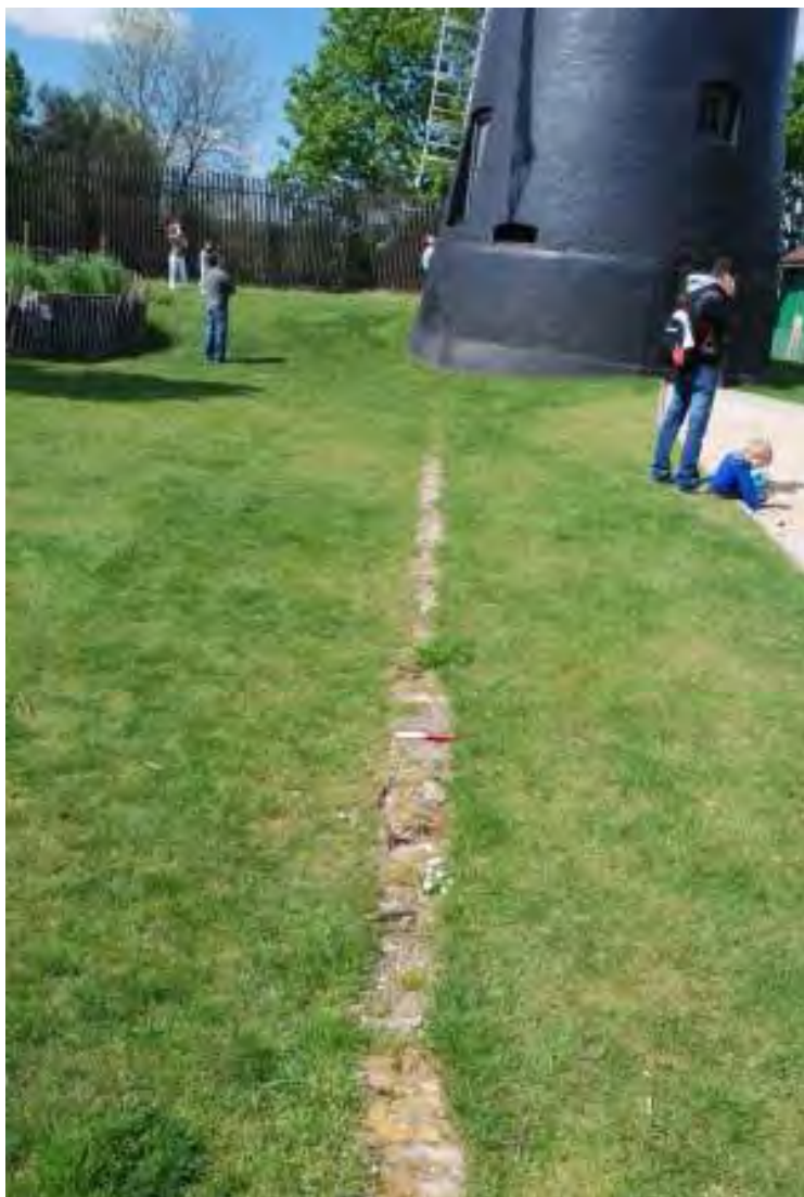
Fig. 32: Line of frogged yellow stock bricks leading to the east from the windmill.
