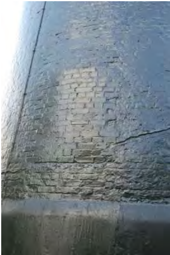
Fig. 39: Photograph of the patched-up brickwork indicating the location of the blocked-up doorway at first-floor level on the northern side of the structure.
