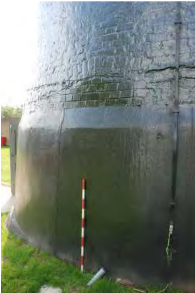
Fig. 36: Photograph of the blocked-up doorway on the northern side of the mill, at ground-floor level.
