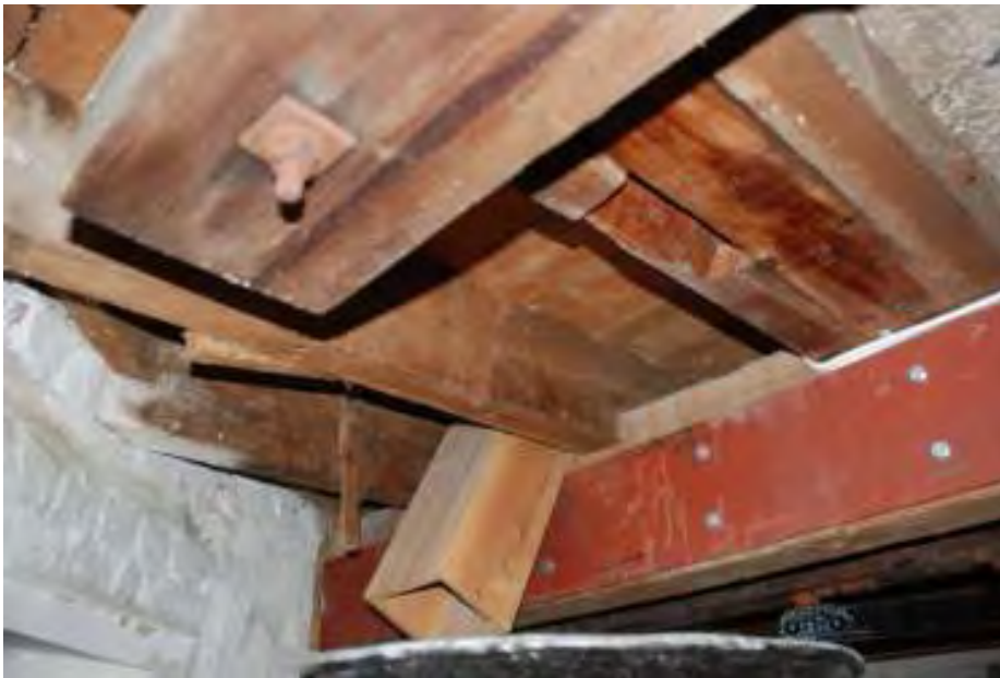
Fig. 86: Photograph of the (replica) wooden chute which would have brought the meal down from the floor above.
