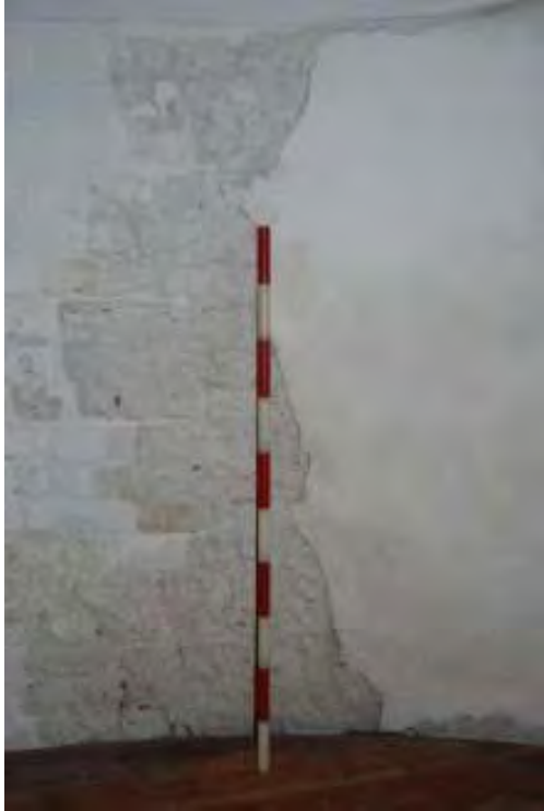
Fig. 54: Photograph of the whitewashing of the interior of the walls, with the brickwork visible behind.
