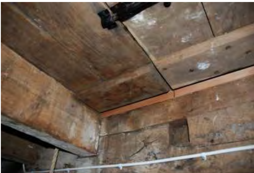
Fig. 60: Photograph of the trapdoor in the ceiling of the third floor, with the empty mortice hole directly beneath it, showing that there had once been an east-west beam here and that this was not the original location of the trapdoor.
