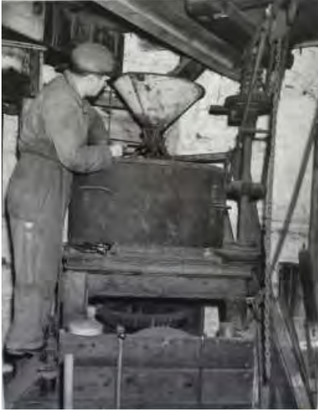
Fig. 22: Photograph of the 1964 restoration works (restoring the millstone frame) (LMA).
