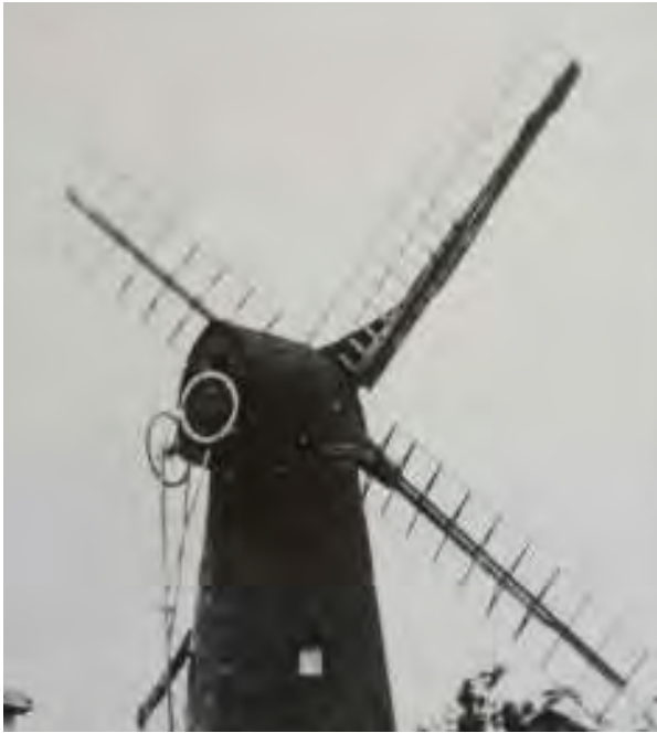
Fig. 48: Extract from a pre-1862 photograph showing the two different types of sails. The top right sail is a patent sail; the top left and bottom right sails being common sails (from Greater London Council 1967 pamphlet).
