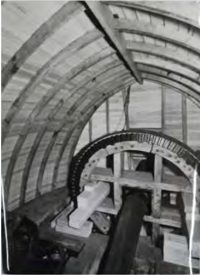
Fig. 28: Photograph of the cap, with windshaft and brake wheel, post-1964 restoration works (LMA).
