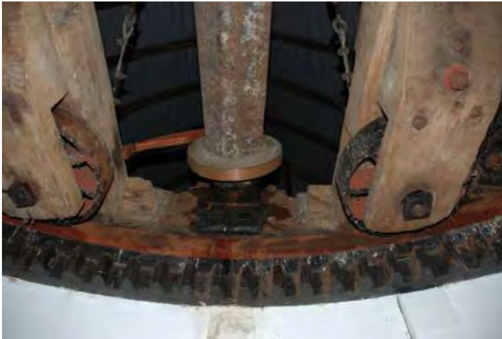
Fig. 65: Photograph of the iron teeth connecting the mill to the cap, and the horizontal wheels which kept the cap in position.
