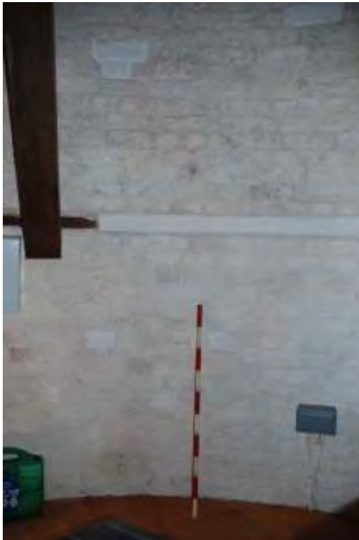
Fig. 55: Photograph of the interior of the windmill, showing the horizontal pieces of timber (above the scale), and occasional replaced bricks.
