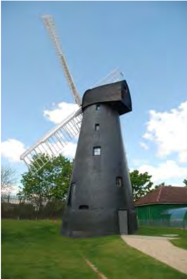
Fig. 41: Photograph of the windows, showing one on the first-floor (on the eastern side, above the present door), and one on the second, third, and fourth floors (on the south-eastern sides of the structure).
