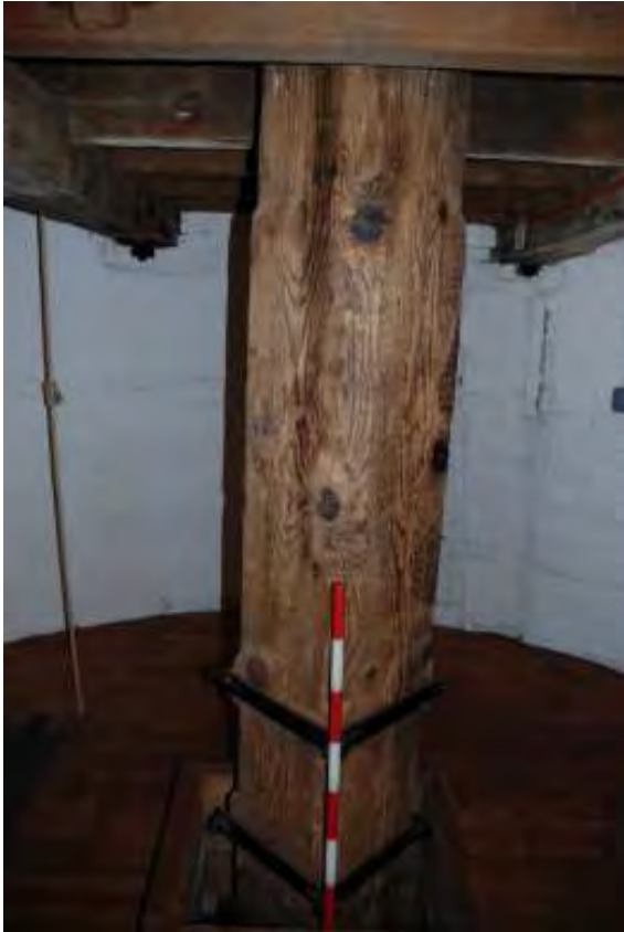
Fig. 67: Photograph of the central vertical shaft, used to transfer the drive down from the sails.
