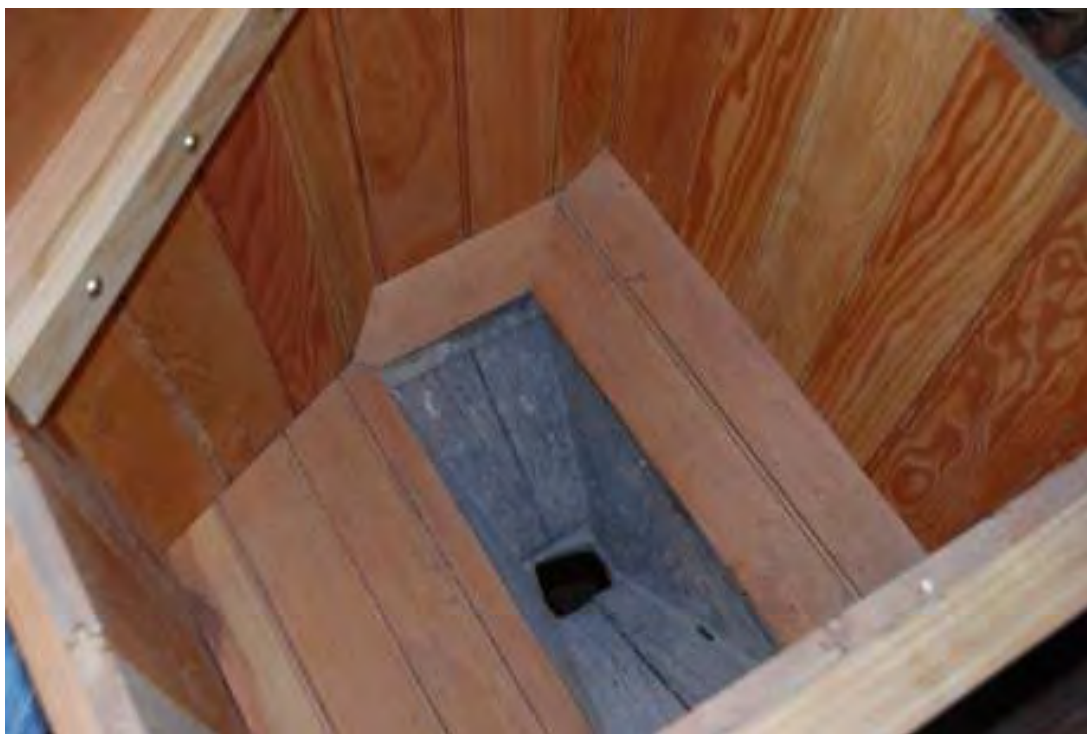
Fig. 76: Photograph of the wooden chute in the north-east corner of the second floor, possibly original.
