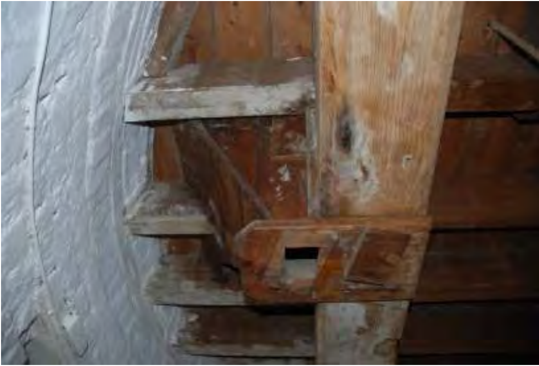
Fig. 78: Photograph of the wooden chute on the north-eastern side of the second floor, leading down from the third floor.
