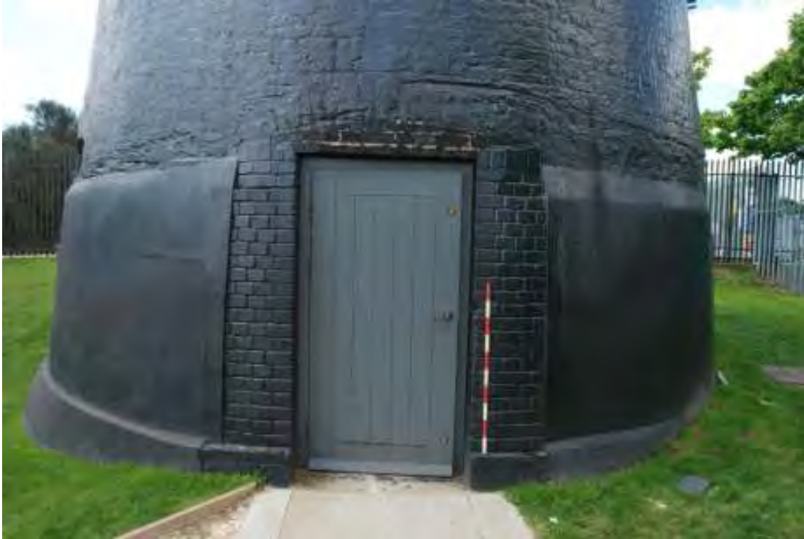
Fig. 31: Photograph of the bottom part of the mill structure (around the present door), showing the additional protective layer of tar, covering two 'steps out' in the base.
