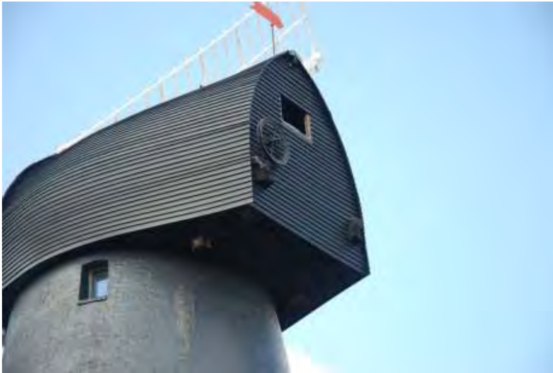
Fig. 44: Photograph of the rear of the cap today, depicting the (replica) wheel which helped operate the patent sails.
