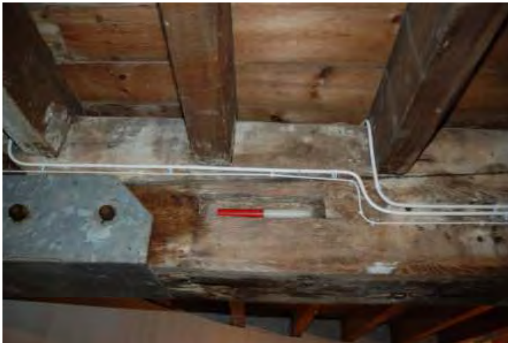
Fig. 93: Photograph of the main east-west beam on the ground-floor, with an empty mortice hole suggesting that this may be a reused beam.
