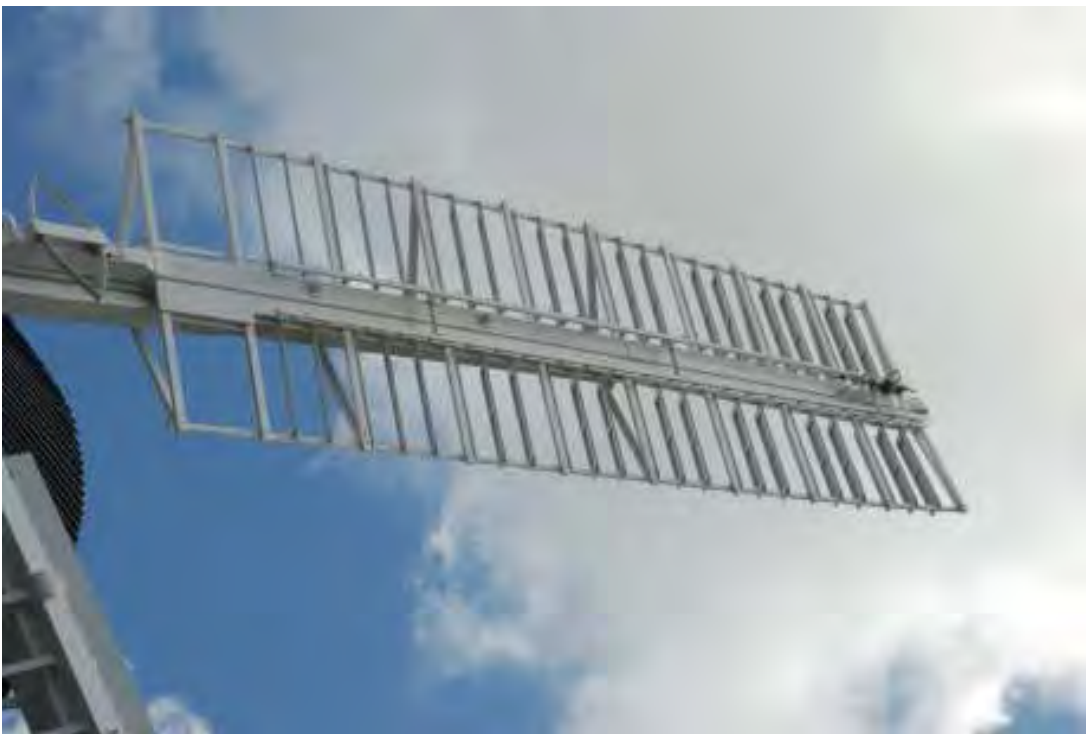
Fig. 50: Photograph of one of the 'patent sails' today. The wooden shutters, which were opened and closed dependent on the wind, can be seen.
