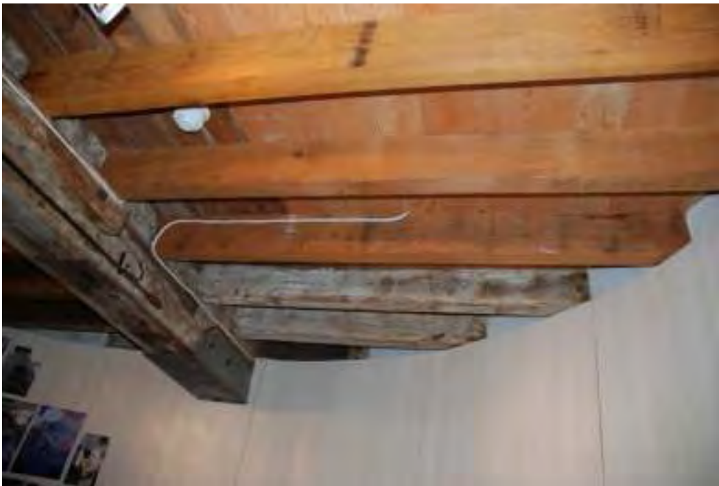
Fig. 56: Photograph of the ceiling beams and floorboards, looking up from the ground-floor. The beams and floorboards inserted during the 2010 renovation works are visible (orange coloured) plus those inserted in the 1960s (far end of frame).
