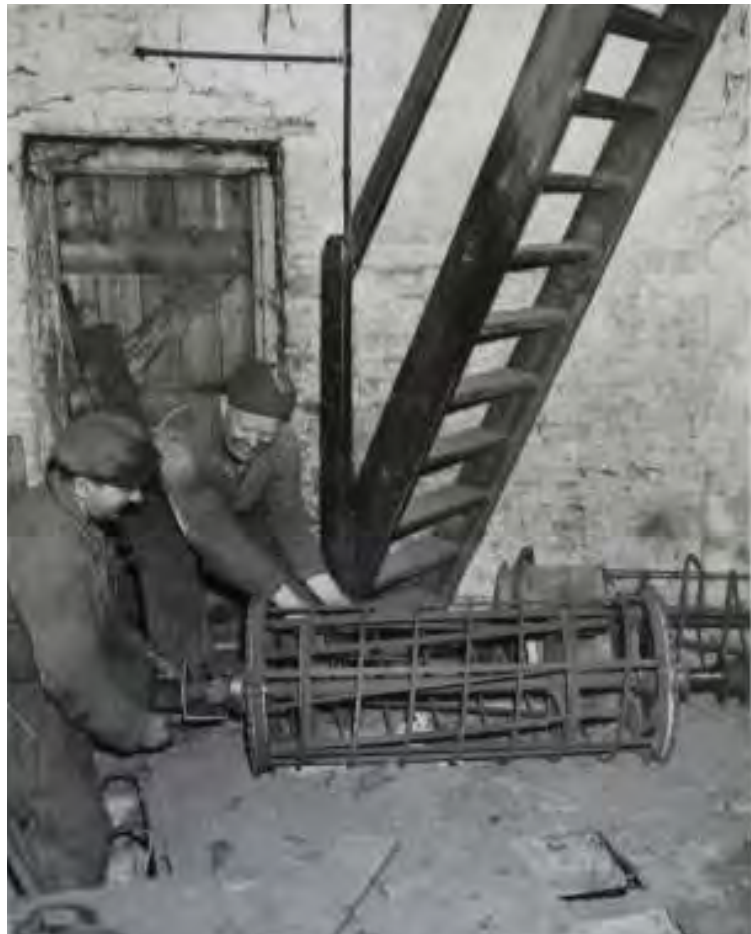
Fig. 23: Photograph of the 1964 restoration works (removing a corn sifter) (LMA).
