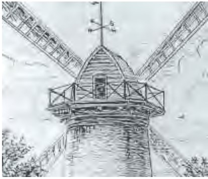
Fig. 46: Extract from a c.1880 image of Brixton Windmill, clearly showing the gallery inserted around the base of the cap (Lambeth Archives, Landmark).
