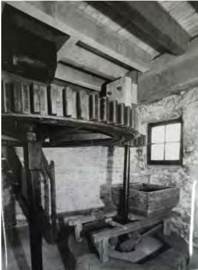
Fig. 27: Photograph of the spur wheel, stone nut, and vat, post-1964 restoration works (LMA).
