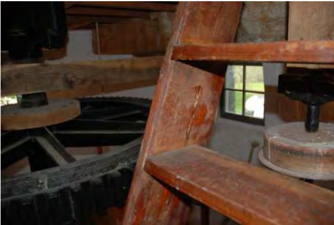
Fig. 75: Photograph of the spur wheel (left of frame) with the smaller wooden wheel above this, which would have been connected to the governor wheel (right of frame).
